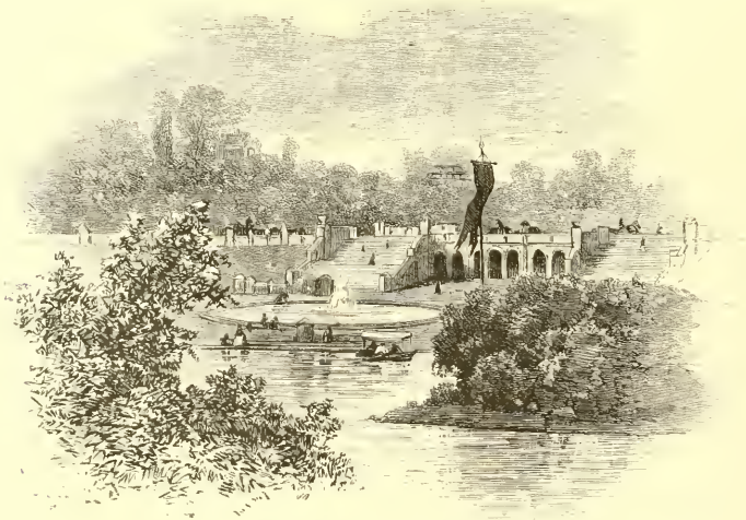
THE TERRACE FROM THE NORTH.
